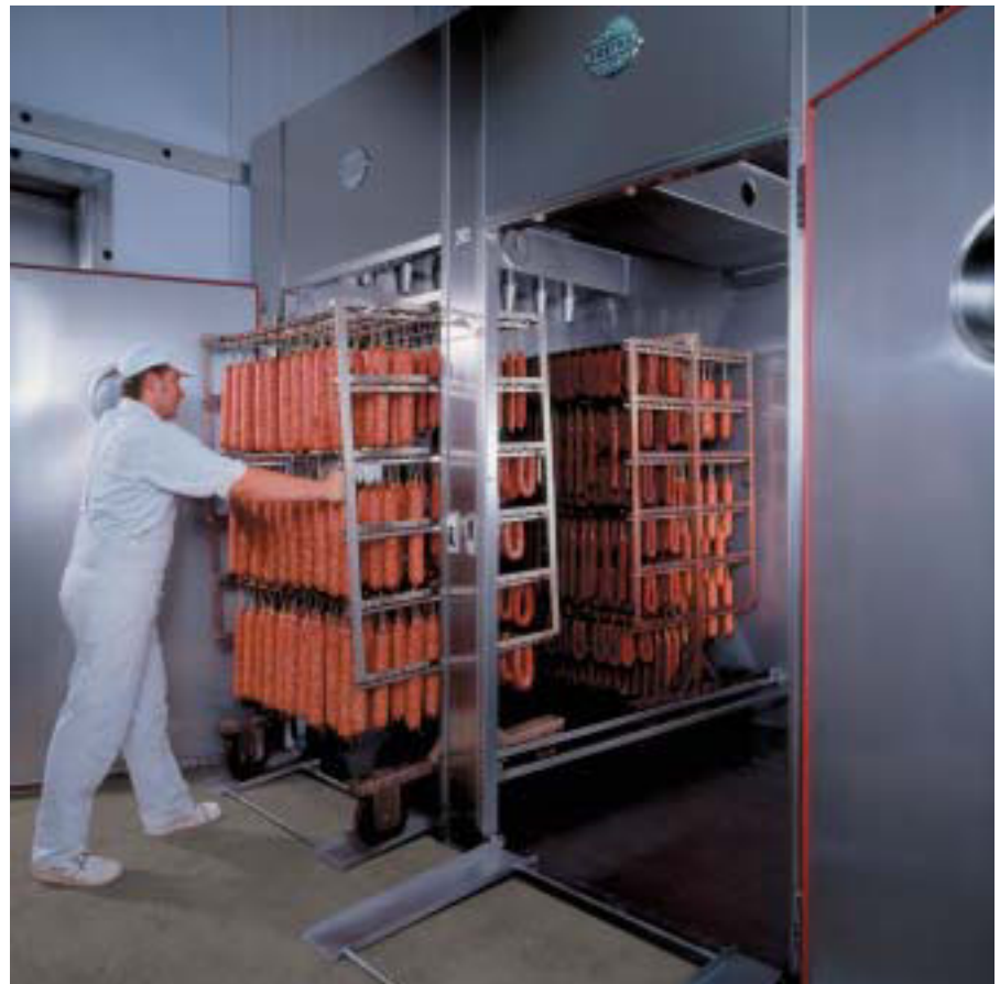
4-truck chamber maturing smoke installation
